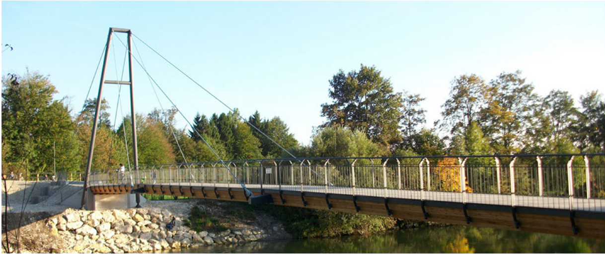
Figure 11. Walkway in Tauberbischofsheim, Germany, 2009. Source: Miebach Engineering.
