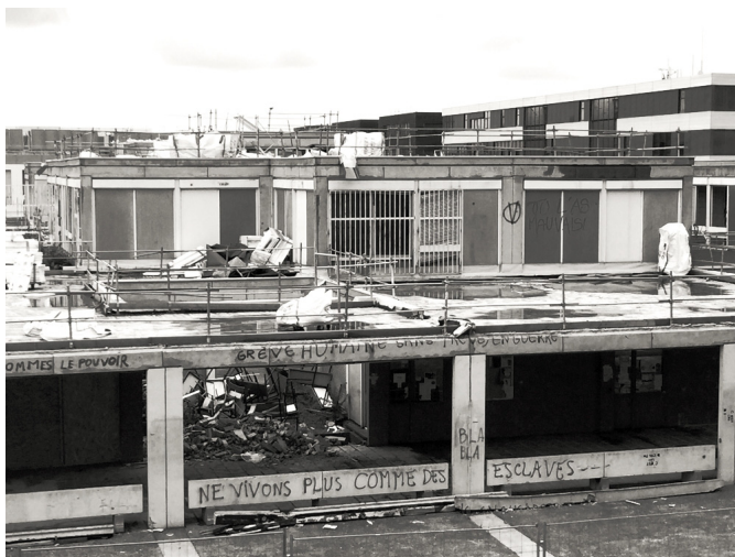
Figure 5 – Toulouse-Le Mirail. Demolition of university buildings in 2016. Source: author’s photograph.
